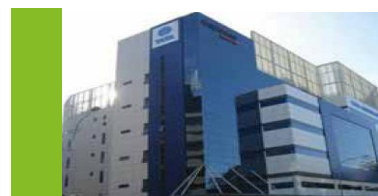
Tata Communications Exchange
